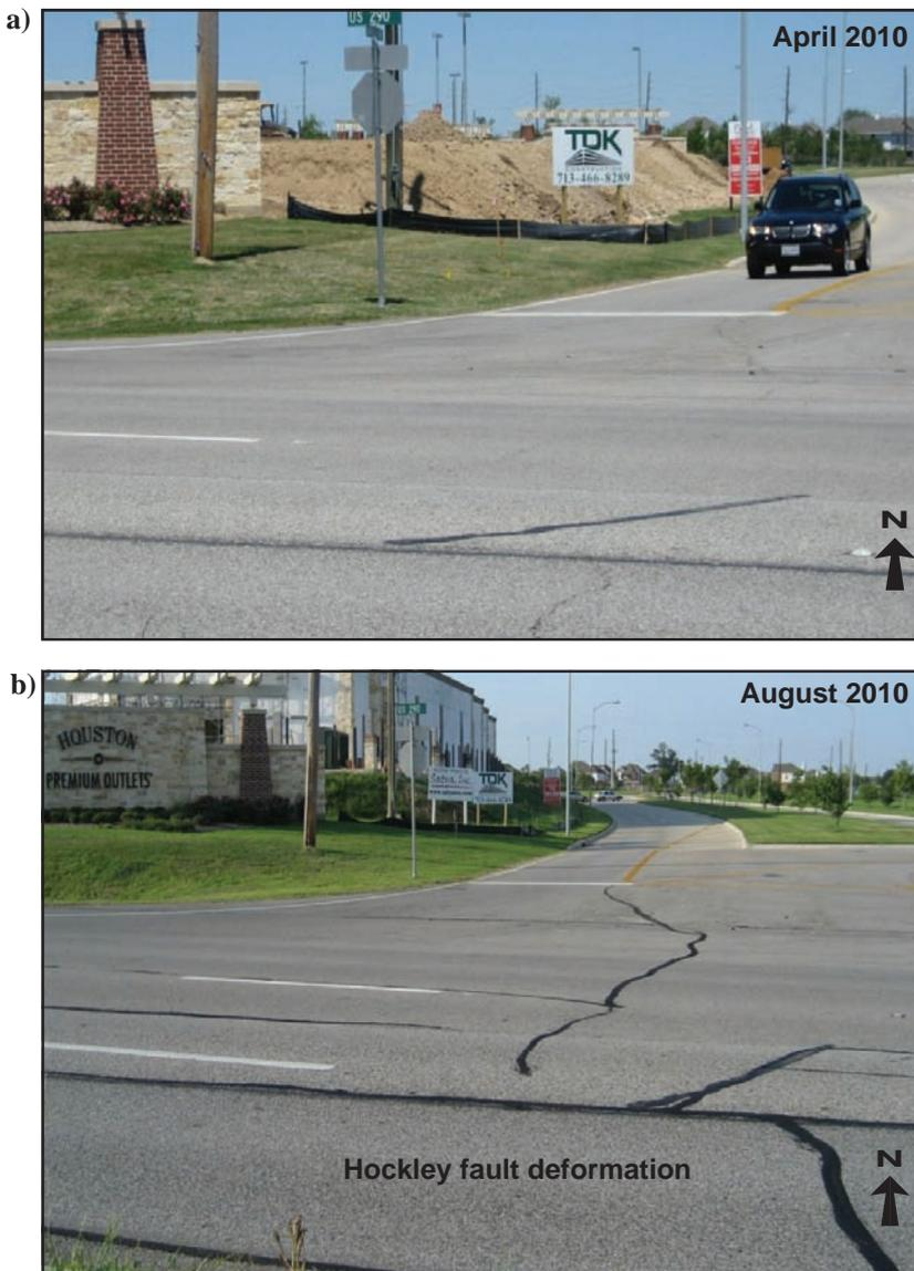
Figure 12. (a) Newly paved asphalt has been placed over the Hockley Fault in April 2010 at the entrance road of the shopping center. Note that this part of the mall was still under construction at that time; (b) the fault deformation manifested itself within three months, and cracks were patched with black asphalt.
