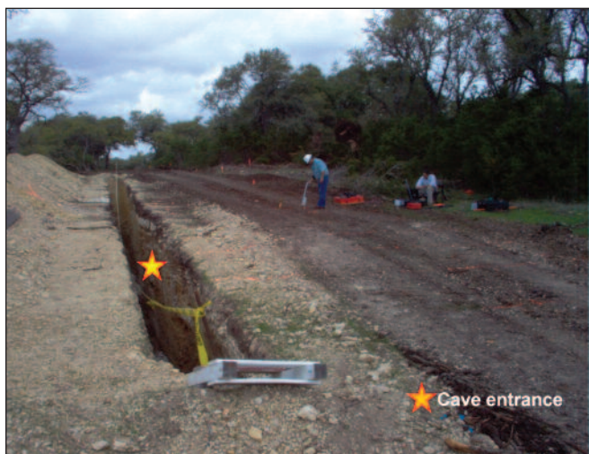
Figure 7 A picture that shows the location of Cave 4 along a trench. The ceiling of the Cave is 12 feet from the surface.
